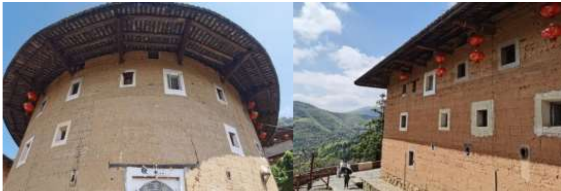
Figure 6. The earth wall of Ruiyun Building & Buyun Building
