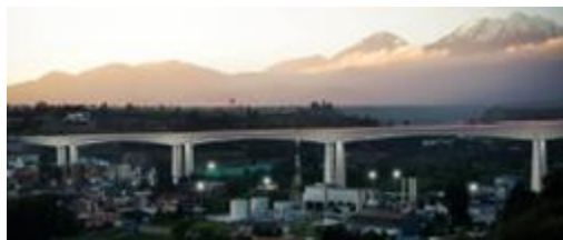
Figure 6. Chilina Bridge in Arequipa
