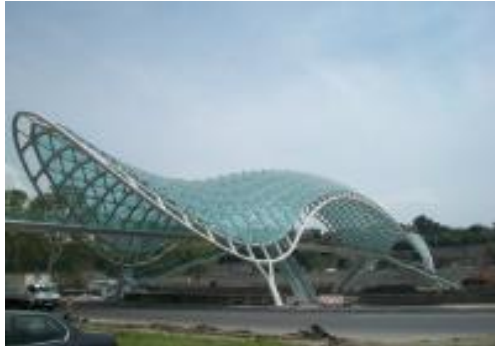
Figure 4. Tbilisi Bridge in Georgia
