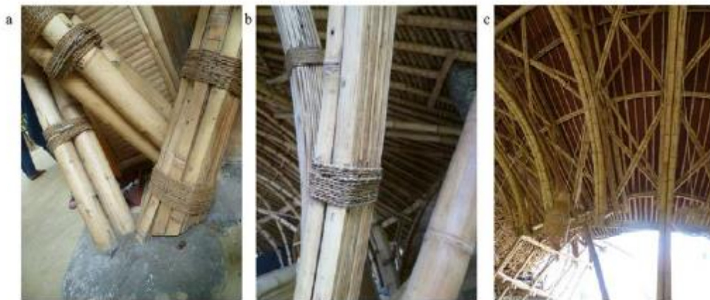
Figure 6. Bamboo connection using Tali
