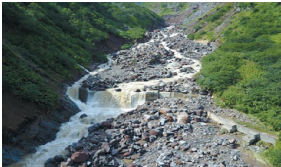
Fig. 1 Stabilization of river bed transformations before a barrage
