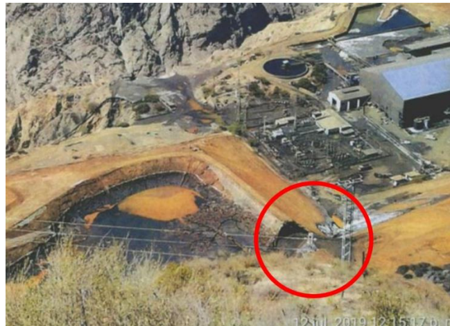
Figure 4. View of the breach in the dam 2 days after the failure in the North Area tailings deposit.
