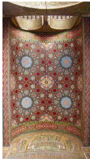
Figure 1. Damascus: Umayyad Mosque, entrance hall ceiling (Source: Author).
