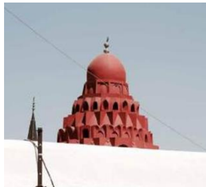
Figure 11. Damascus: Al-Madrasa al-Nuriyya al-Kubra, 1167. The exterior of the muqarnas dome (Source: Author).
