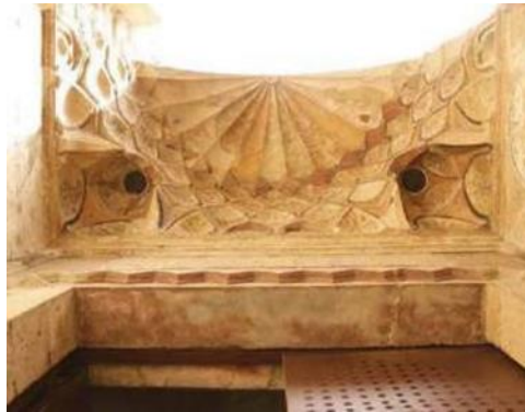
Figure 17. Damascus: Eastern entrance of the Citadel, 1214. Looking up at the muqarnas (Source: Author).
